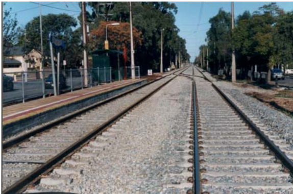
Photo – Section of Upgraded Tramline at Forestville
