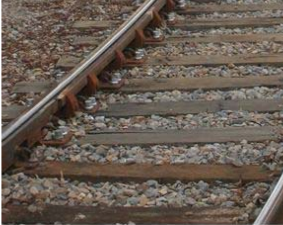
Figure 19 – Bar-Type Checkrails
