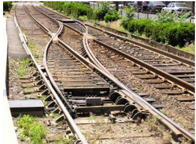
Figure 10 - Blade Protection Measures Adopted in Boston
