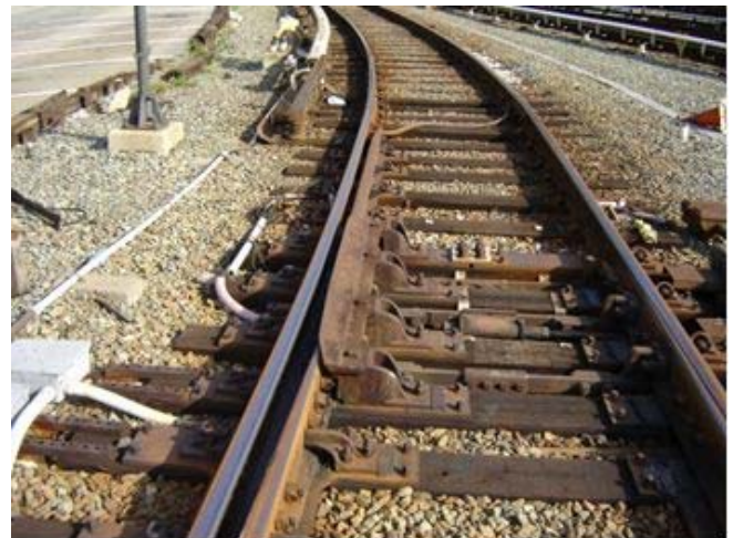
Figures 11 – Blade Protection Measures Adopted in Washington
