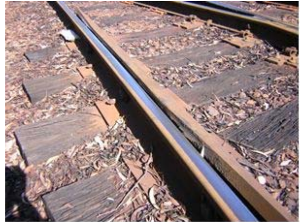
Figure 4 - Wear on Checkrail
