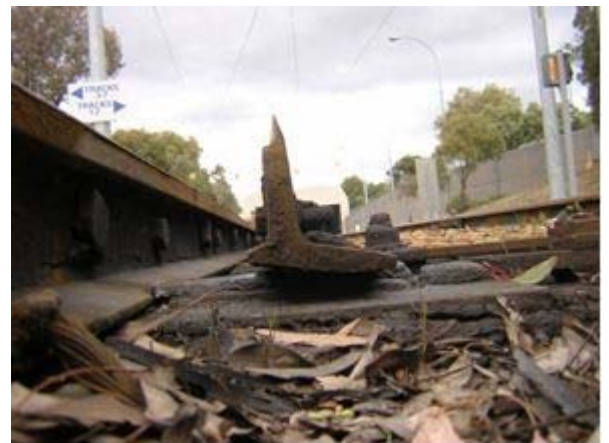
Figure 5 – Form of Existing Switchblade
