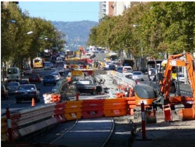
Photo – View of Trackwork on North Terrace
