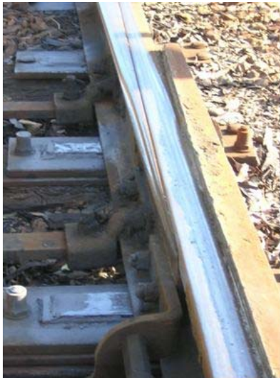
Figure 7 – Wear in Blade
