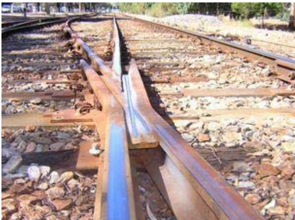
Figure 3 – Infilled V-Crossing
