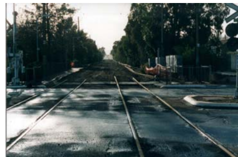
Photo – Track Removed at Forresterville
