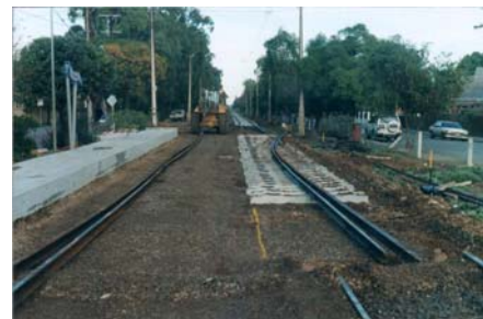
Photo – Track being Laid
