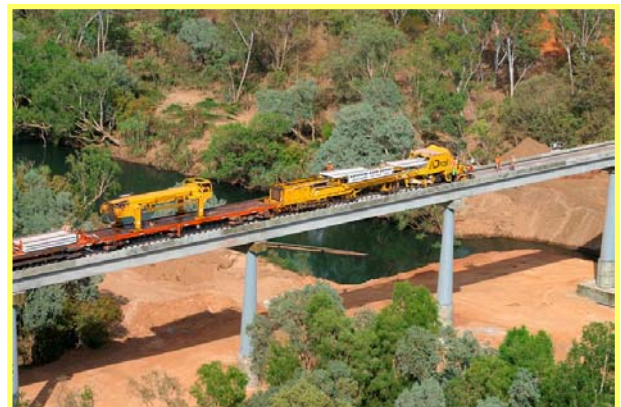
Tracklaying Across the Katherine River Bridge – Sept 2002
