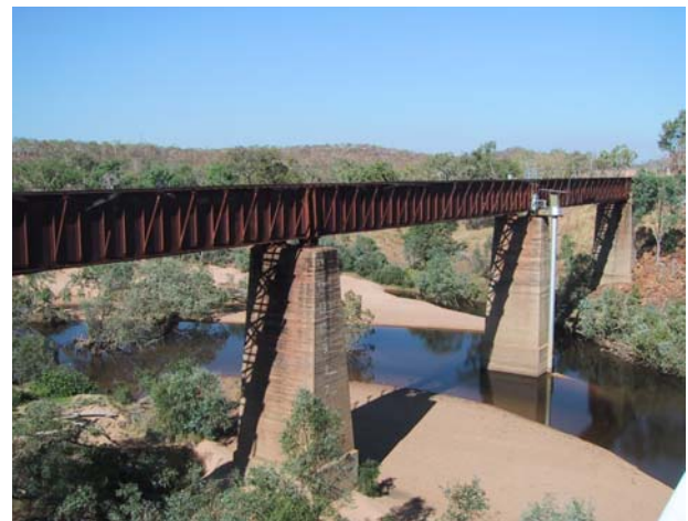
Ferguson River Bridge
