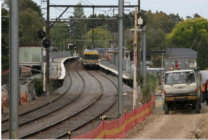
Old Laburnum station prior to the shut down showing the reverse curves and 1 in 40 grade. This station was the scene for more traction motor failures than any other place on the network back in the days of Tait and Swing door trains
