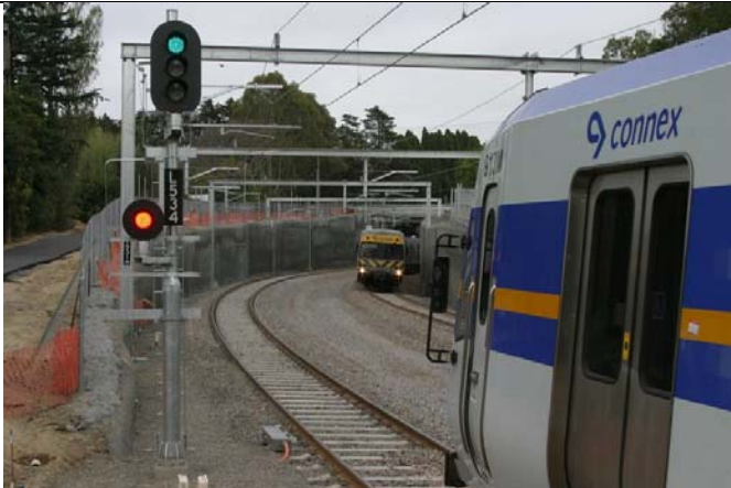
A view from the up end of Laburnum station after resumption of services looking into the cutting toward Middleborough Road bridge (visible above the approaching Comeng train).
