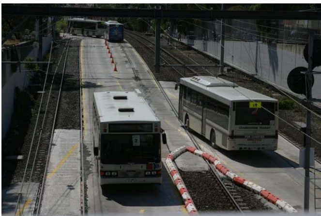
The bus road into Box Hill station. Note the 'wrong road' working. The only difficulty with the buses was the lack of co-operation by the VicRoads crowd who failed to manage traffic light operation properly to keep the buses flowing smoothly.
