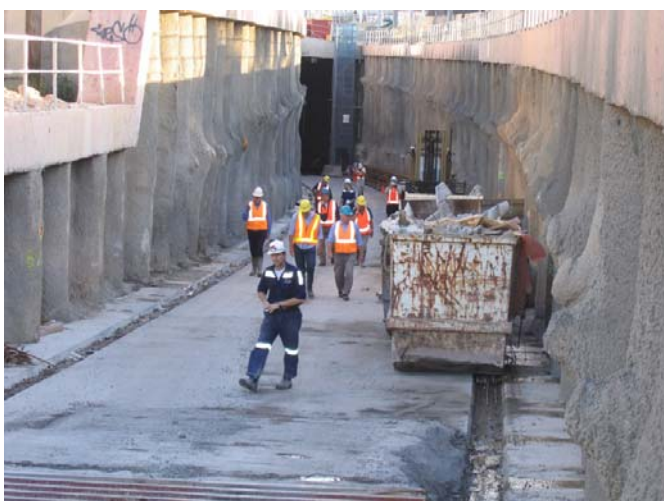
Walking wrong-road up the Epping Up Ramp
