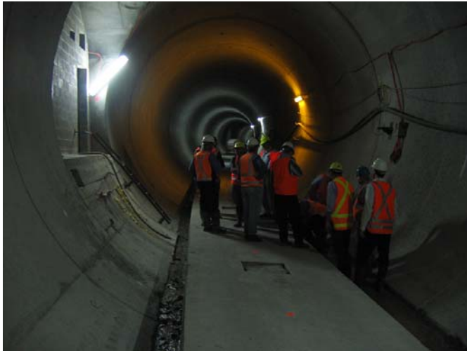
Floating slab successfully passes the Engineer Loading Test
