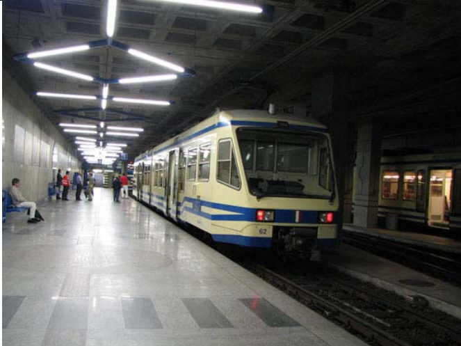
Locarno SSIF station is a quite elaborate underground affair
