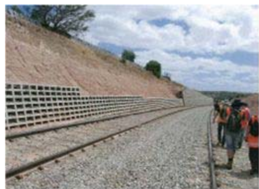
Track Upgrade including Embankment Stabilisation and Drainage
