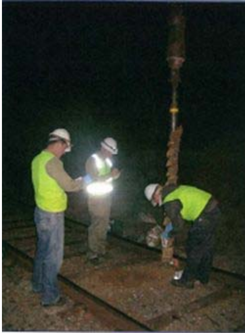
Geotechnical Investigation on the Belair Line
