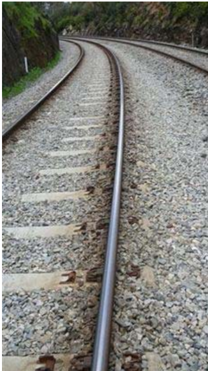
Upgraded Track on the Belair Line
