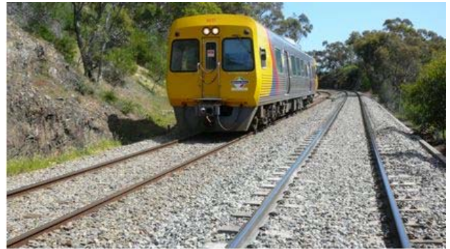
Track Upgrading on the Belair Line
