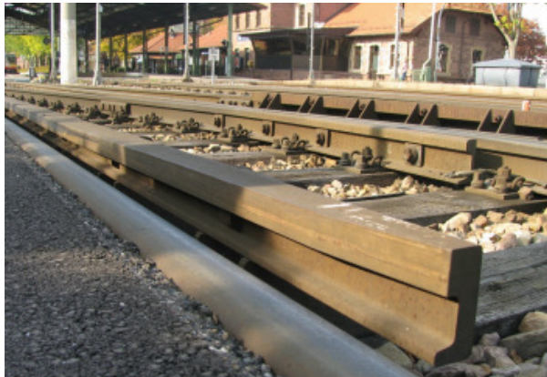
A standard raised check rail on German railways, 20 mm – 40 mm above running surface (Karlsruhe)
