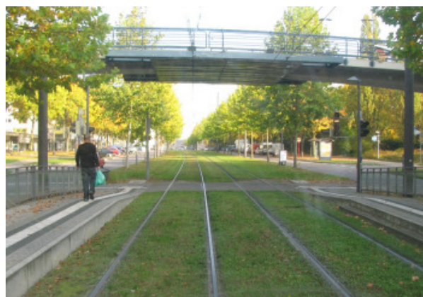
Urban corridors are typically very wide and are used for infrastructure of economical size (Karlsruhe)
