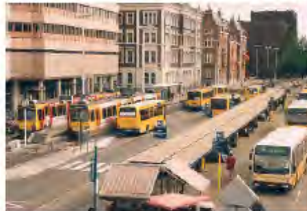
Fast Bus and Tram Interchange
