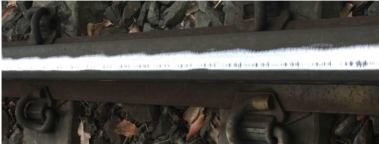
Figure 1 Typical rail head with the once-per-revolution longitudinal roughness evidenced by the thickness of the region worn by passing wheels
