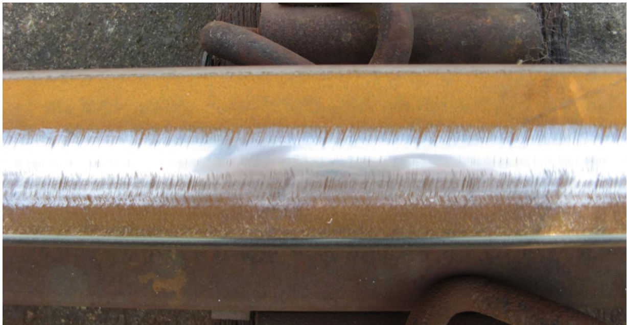
Figure 2 Newly ground rail after several weeks of traffic
